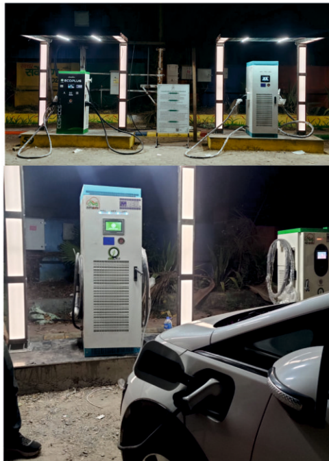
EV chargers Live at Mai Mangeshkar site in Indore with GB/T gun and CHAdeMO gun converted into CCS-II gun.
