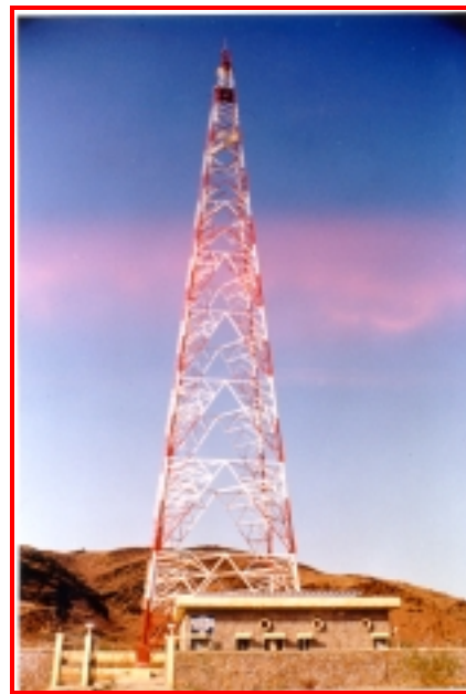
MICROWAVE REPEATER STATION AT SAWAI MADHOPUR
